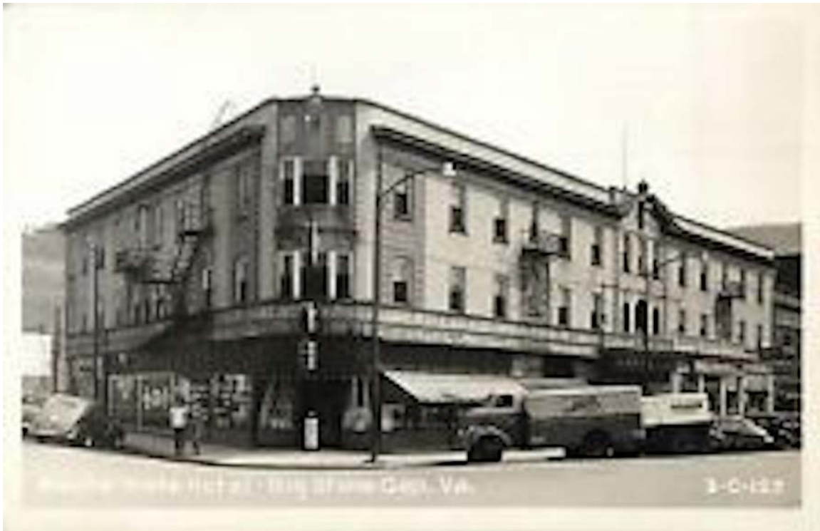
THE MONTE VISTA HOTEL ON THE CORNER OF E. 5 TH STREET AND WOOD AVE. IN THE CENTER OF BIG STONE GAP, VA. – KELLY DRUG OCCUPIED THE PROMINENT FIRST FLOOR CORNER – THE SEVERAL LAW OFFICES MENTIONED WERE IN THE SAME BLOCK TO THE RIGHT
